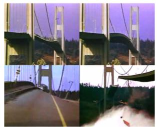
Fig. 1 Collapse of Tacoma Narrows Bridge [2].
